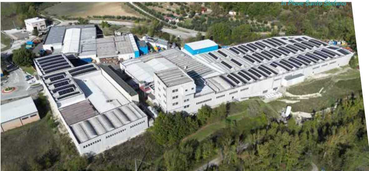
Photovoltaic panel installation at Tratos HV
