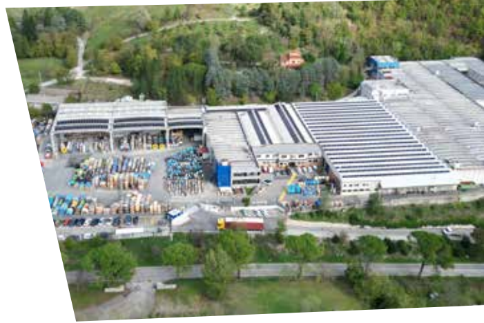
Photovoltaic panel installation at the Tratos Cavi plant in Pieve Santo Stefano
